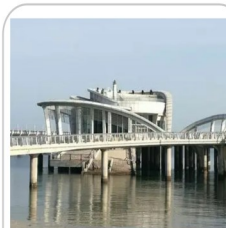
Pegasus Trestle Bridge
